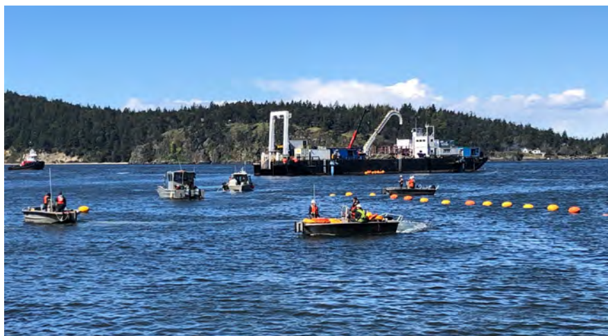
A team of specialized crew installing submarine cables in Active Pass.
