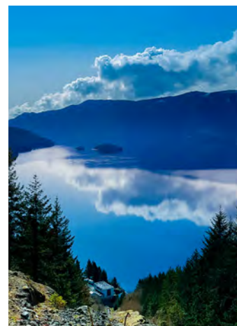
Ash River Generating Station is an important resource that contributes about 6% of BC Hydro's Vancouver Island hydroelectric generation.
