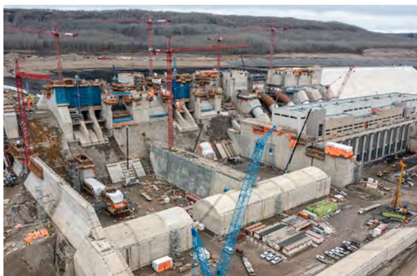
This aerial view shows Site C's spillways, penstocks, powerhouse and operations building for BC Hydro's third dam along the Peace River.
