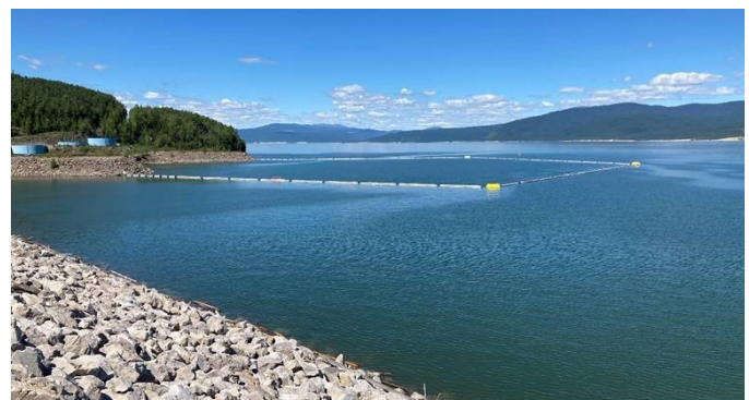
New boom made of galvanized steel
