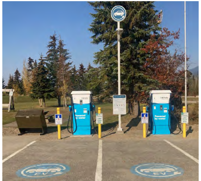
The recently upgraded electric vehicle fast charging site in McBride. Photo courtesy of: BC Hydro Media Relations.
