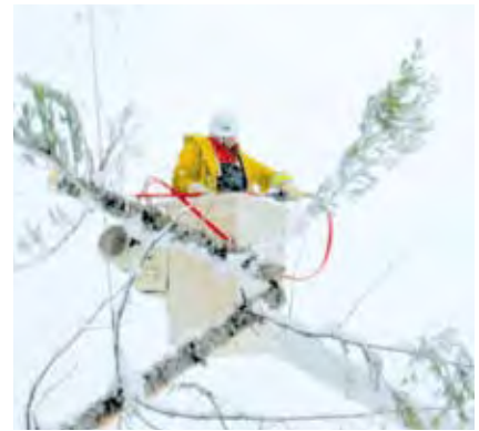
Power line technician during a Campbell River snowstorm.
